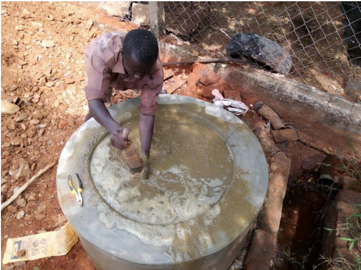
Picture 4: showing Training to a gardener on how to mix the cow dung before release it in the digester
