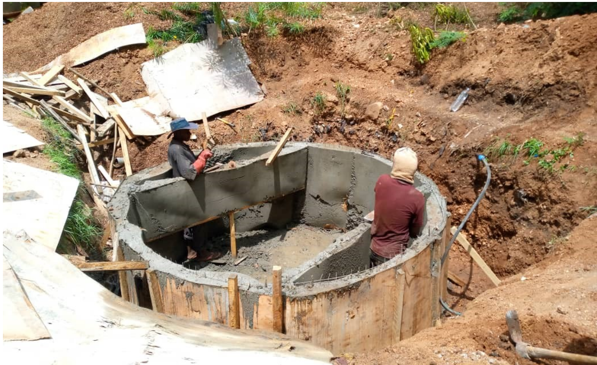
Picture 1 &2: showing the construction of the biodigester system at DB Oysterbay.
