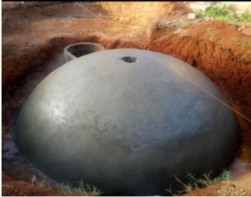
Picture 3: showing the constructed of the biogester system at DB Morogoro
