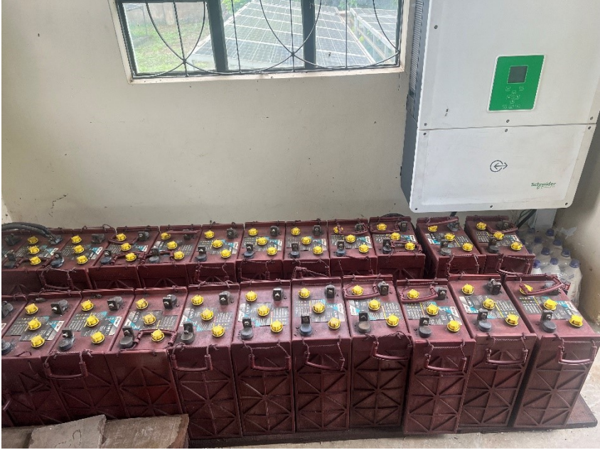
Photo 2; Showing the old lead-acid batteries, which have been replaced.
