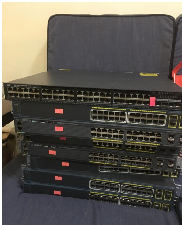
Picture 1 Showing the CISCO switch catalyst 2960 POE purchased items before installation.
